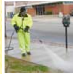
Power washing Downtown sidewalks
